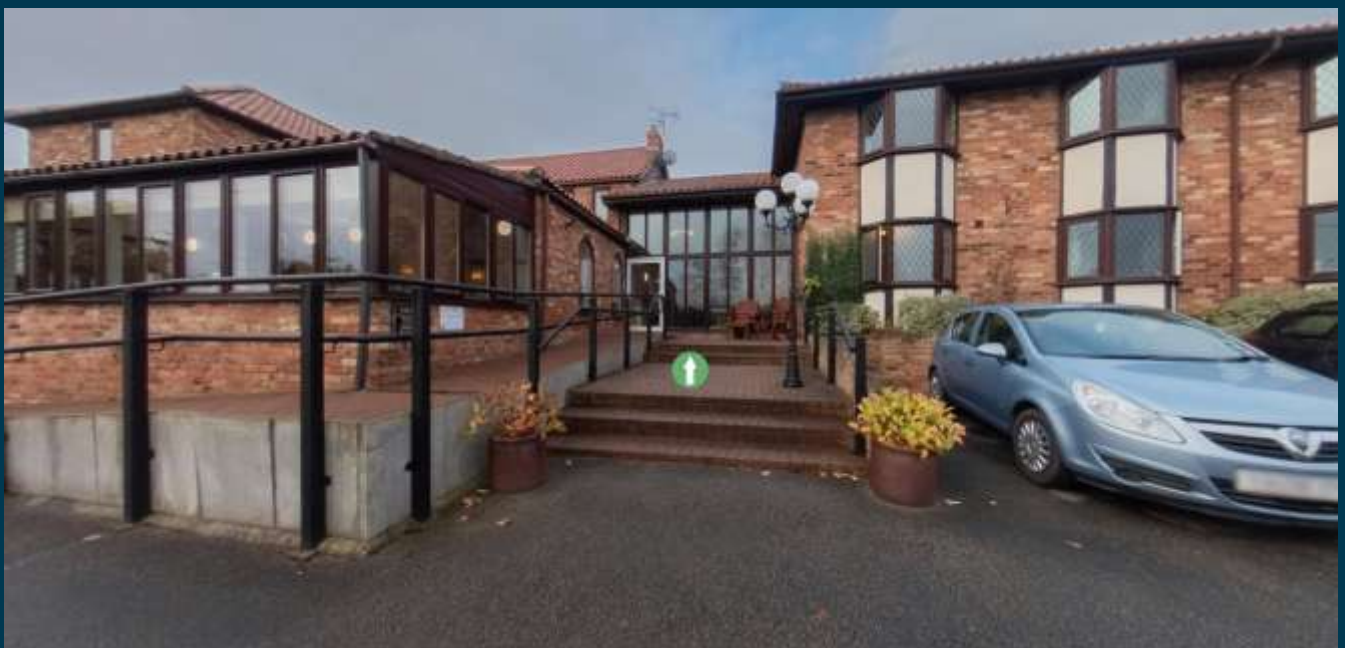
Riverside Care Complex
